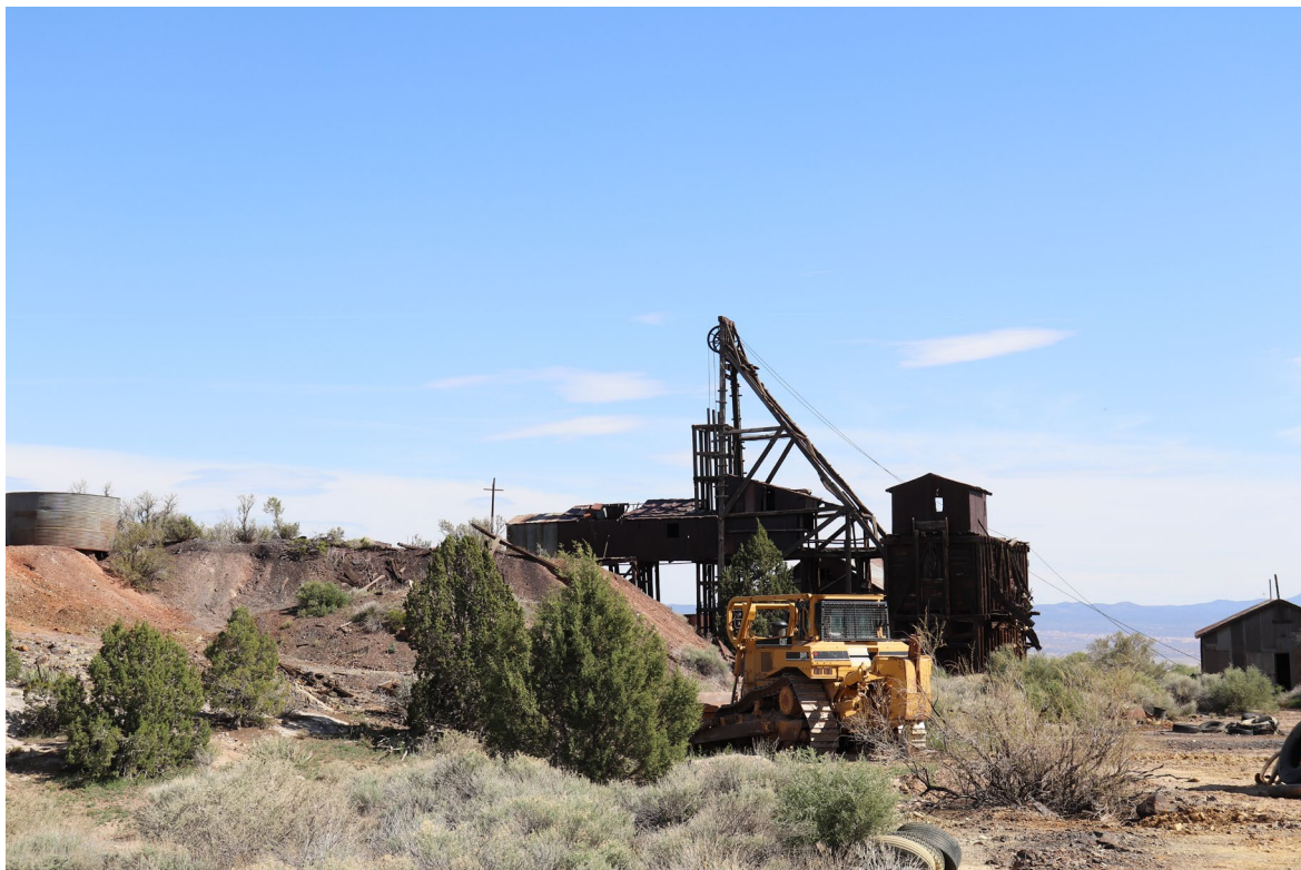
Mining headframe from previous production on the property
