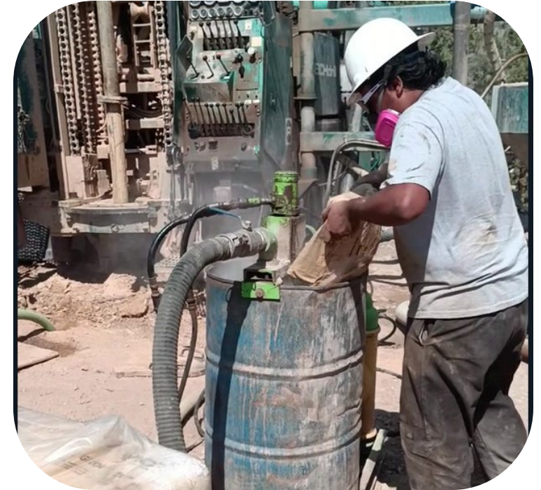
Closing a completed hole
